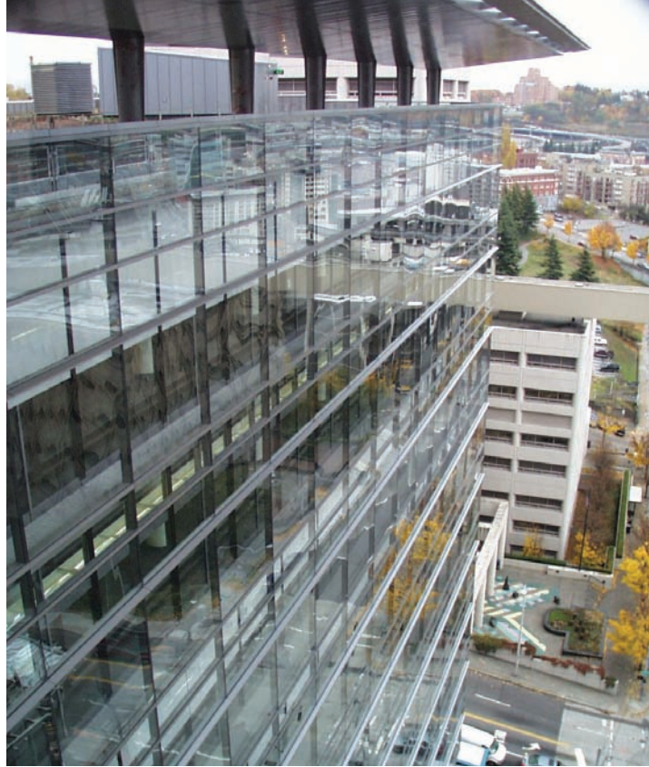
The 300,000-square-foot, $69 million Seattle Justice Center was built in 2002 and awarded a LEED Silver Certification by the U.S. Green Building Council. The building's features include an energy-efficient lighting system, electronic timer switches, occupancy sensors, and daylighting controls.
