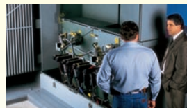
COOPER Power Systems
