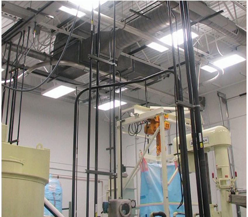
Photo 1. Steel conduit provides unsurpassed protection from conductor damage, however, sales volume dropped by 15% between 1994 and 2004.
